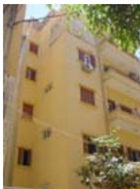
Figure 10.4 Residential building 2: view 2
