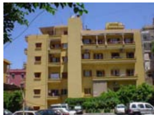
Figure 10.5 Residential building 2: view 3
