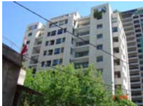
Figure 10.2 Residential building 1: view 2
