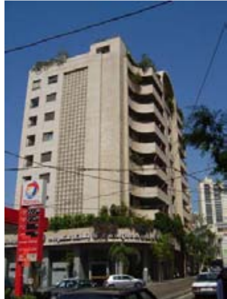
Figure 10.1 Residential building 1: view 1
