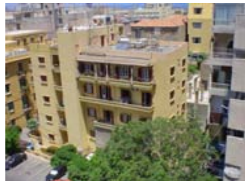
Figure 10.3 Residential building 2: view 1
